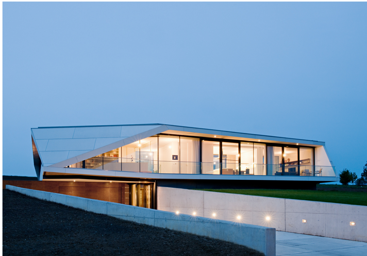
Nordwestansicht Northwest View
