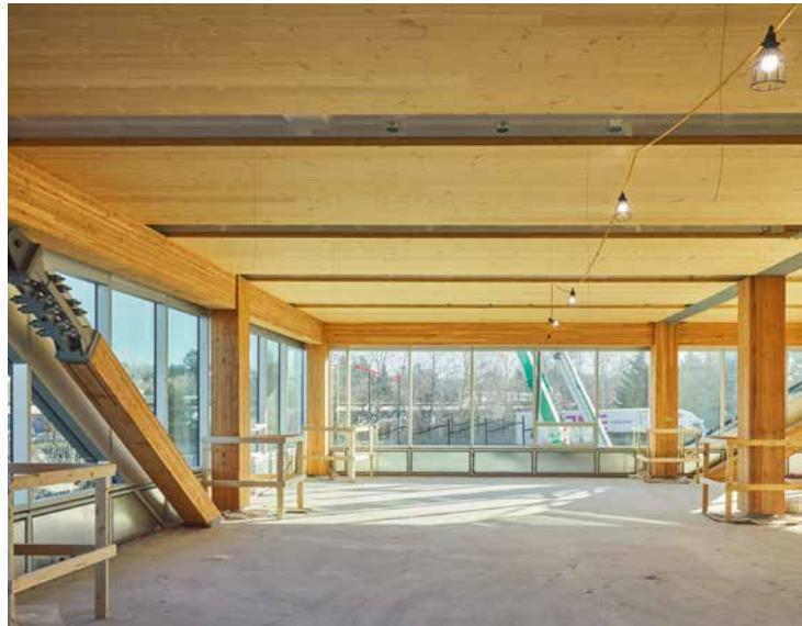
**S**oaring nearly 45 metres above Vancouver, British Columbia's False Creek Flats, The Hive is a 10-storey mass timber office building distinguished by its honeycomb-like façade—a direct expression of its innovative perimeter-braced seismic system. The design features diagonally oriented glue-laminated timber (glulam) braces arranged in a cellular pattern that wraps continuously around all elevations, eliminating the need for conventional cast-in-place concrete cores.
