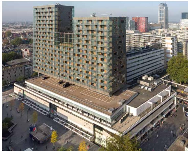
A six-storey Rotterdam retail building from the late 1940s was preserved, rehabilitated and topped with 16 floors of homes, contributing to the repopulation of the city centre. With lightweight hybrid mass timber and steel construction, De Karel Doorman used the existing structure's columns and foundations without compromising structural integrity. The addition is distributed over seven adjoining floors, topped by a nine- and six-storey tower.
