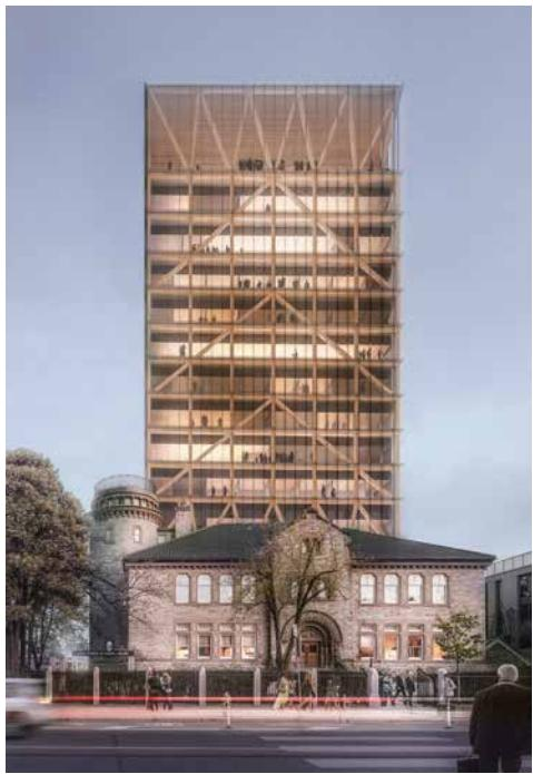
Located along the busy Bloor Street corridor, the University of Toronto's Academic Wood Tower footprint is built on top of the Goldring Centre for High Performance Sport. The north façade of the tower is fully glazed, revealing its mass timber structure to passersby.
