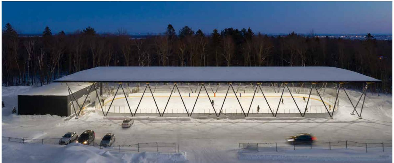
A hybrid design of mass timber and steel creates a roof over an outdoor ice rink that appears to float. Located in a wooded area-turned-city-park in Boischatel, Quebec, Patinoire couverte du parc des Saphirs (Domaine du Boisé) features a roof consisting of 12 glue-laminated timber beams with heights ranging from just over half a metre in the centre to 1.2 metres at the support, tapering again at the outside ends.
