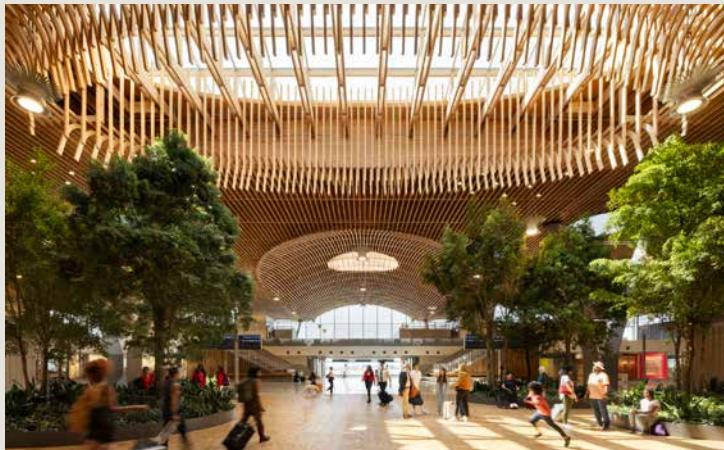
Oregon's **Portland International Airport Main Terminal** in the United States uses layered wood elements to reduce stress and improve spatial clarity. The expansive 36.4-hectare ceiling is made of thousands of Douglas-fir timbers woven into a gently curving lattice that creates soft, wave-like forms overhead. Steel Y-columns rise into this structure at regular intervals, providing both support and a steady visual rhythm. This nested order brings a sense of calm and coherence to the large space.
