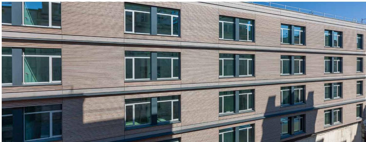
As part of a broader modernization effort, the University Hospital Vienna and the Medical University of Vienna commissioned a new five-storey South Ward Building using modular mass timber. Built on the hospital's joint campus, the facility enables critical upgrades to existing wards without interrupting patient care. The new alternative accommodation meets all structural and building physics requirements for permanently approved buildings.
