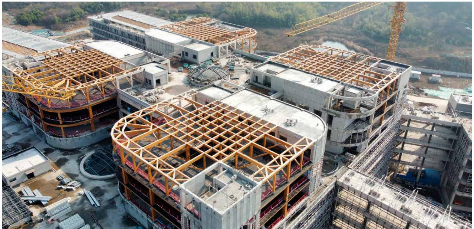
The eight-storey, 208,000-square-metre Jiangsu Provincial Rehabilitation Hospital integrates mass timber and concrete to balance seismic resilience, material efficiency and sustainability.
