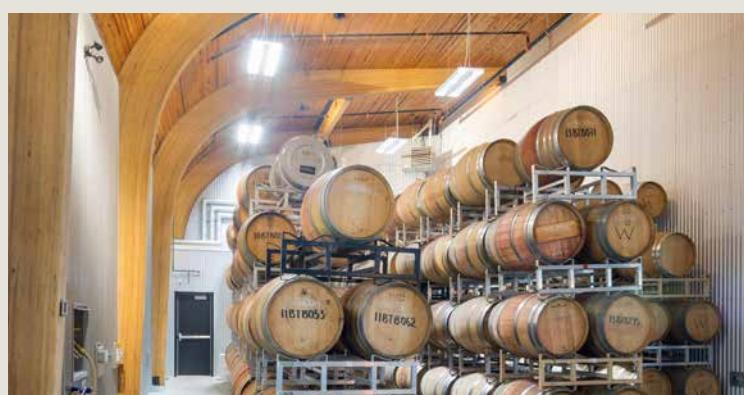
In Penticton, British Columbia, Canada, a 1,670-square-metre former movie theatre has been converted into the **TIME Winery**. The original theatre was built with curved glue-laminated timber (glulam) beams and a nail-laminated timber roof, but was hidden behind acoustic panels and drywall. Three of the former screening rooms have been converted into the winery's state-of-the-art production facility. The fourth has been renovated and kept as a screening room, a reminder of the site's legacy.
