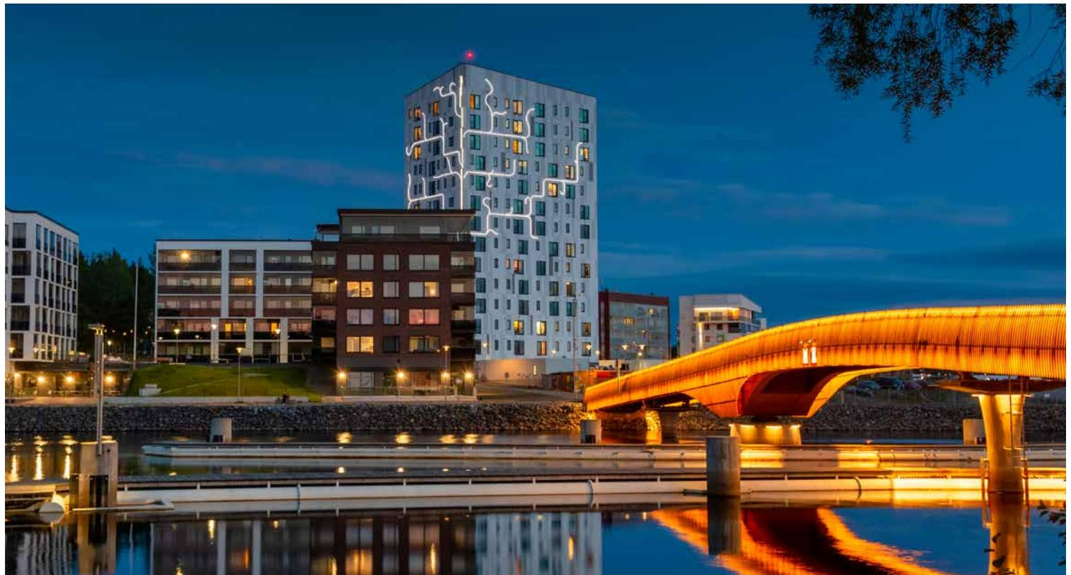
The 14-storey hybrid mass timber Lighthouse Joensuu provides much-needed student housing at the Karelia University of Applied Sciences. The building has 117 one- or two-bedroom apartments across floors two to 14. The ground floor has amenities, including a sauna, laundry room, technical facilities and storage.
